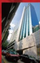
西洋會所大廈(現貌) Club Lusitano Building 1966 - 1978
